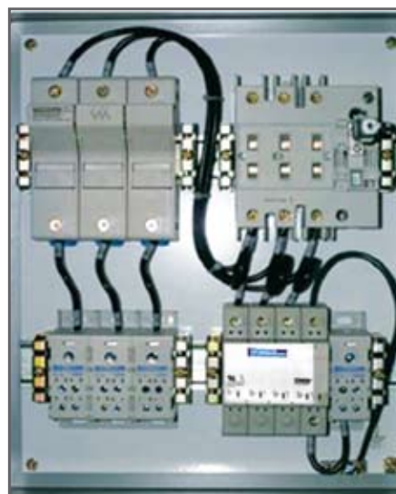
Surge-Trap applied in an electrical panel.
