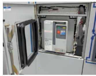
Bellows and Two-Point Door Latch
