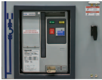
Strengthened One-Piece Breaker Door
